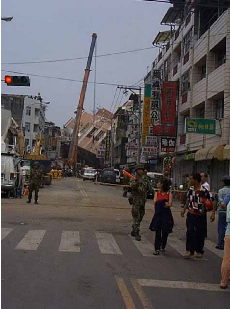
Photograph of Chi Chi earthquake damage 1999 from http://www2.rcep.dpri.kyoto-u.ac.jp
